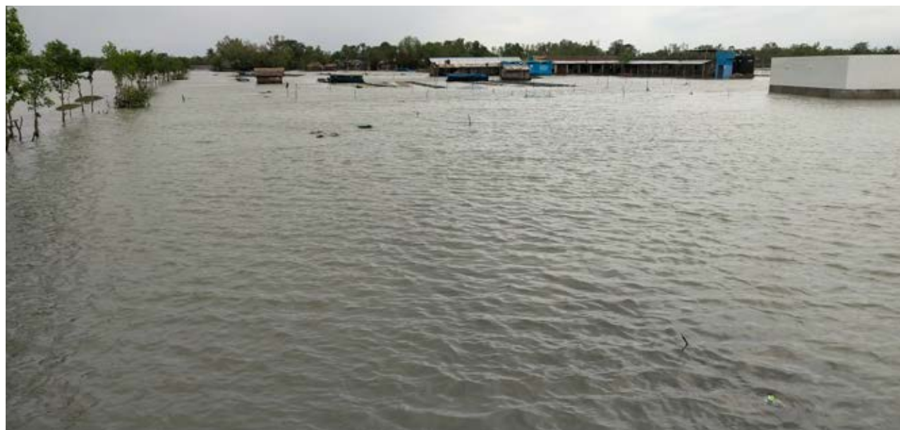
The embankment protecting the Vamia village along the Chuna River collapsed.
