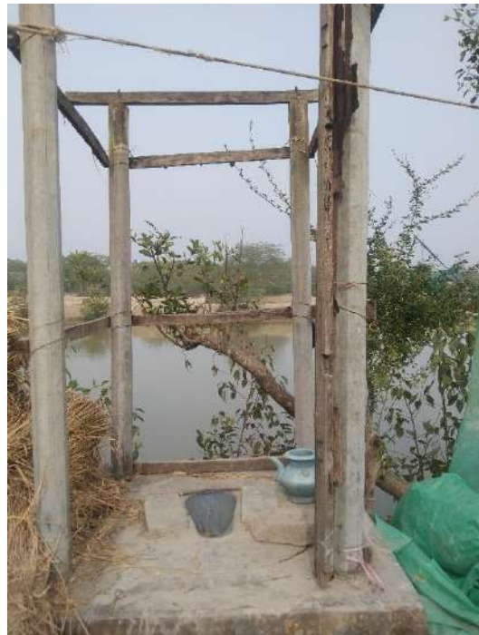
Figure 22: Unsafe and unhygienic latrine of a household in Gabura union (Photo: Author)
