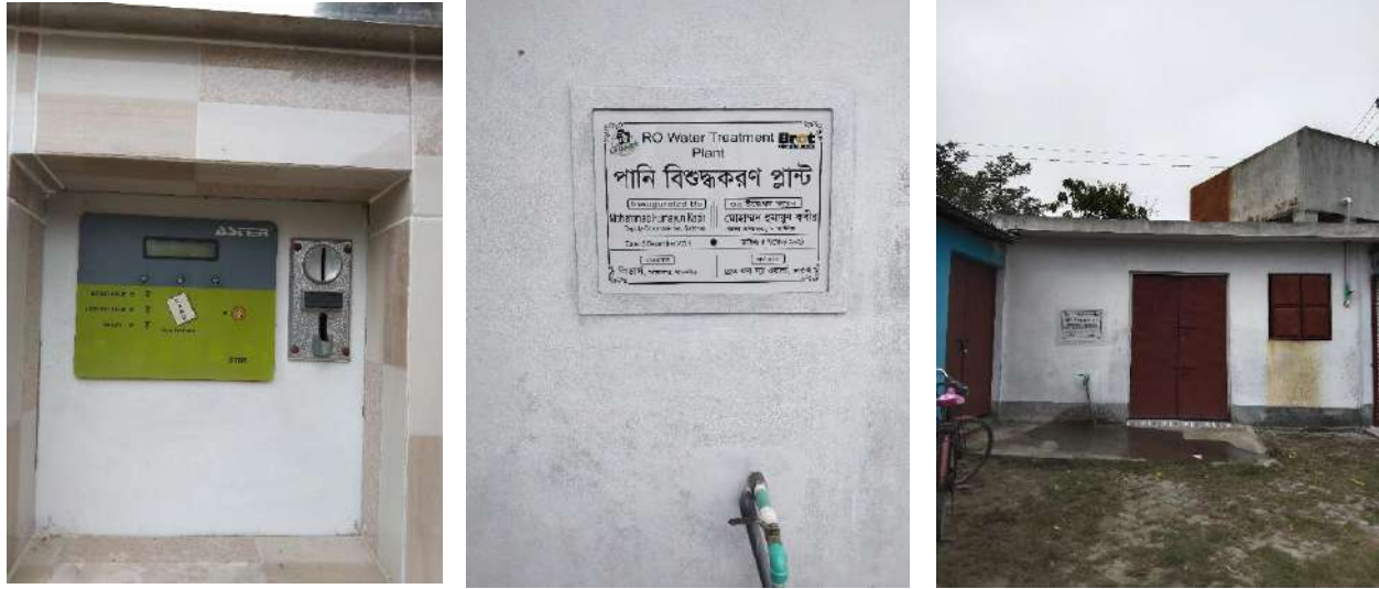
Figure 26, 27 & 28: Freshwater collection booth through rechargeable card system and water treatment plant by LEDARS (Photo: Author)
